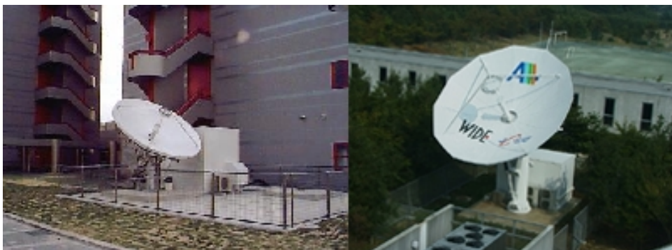
図 2.2 AI 3 Hub Stations located in Japan: The left hub station is for Ku-band located in NAIST and the right one is C-band hub station located in SFC, Keio Univ.
